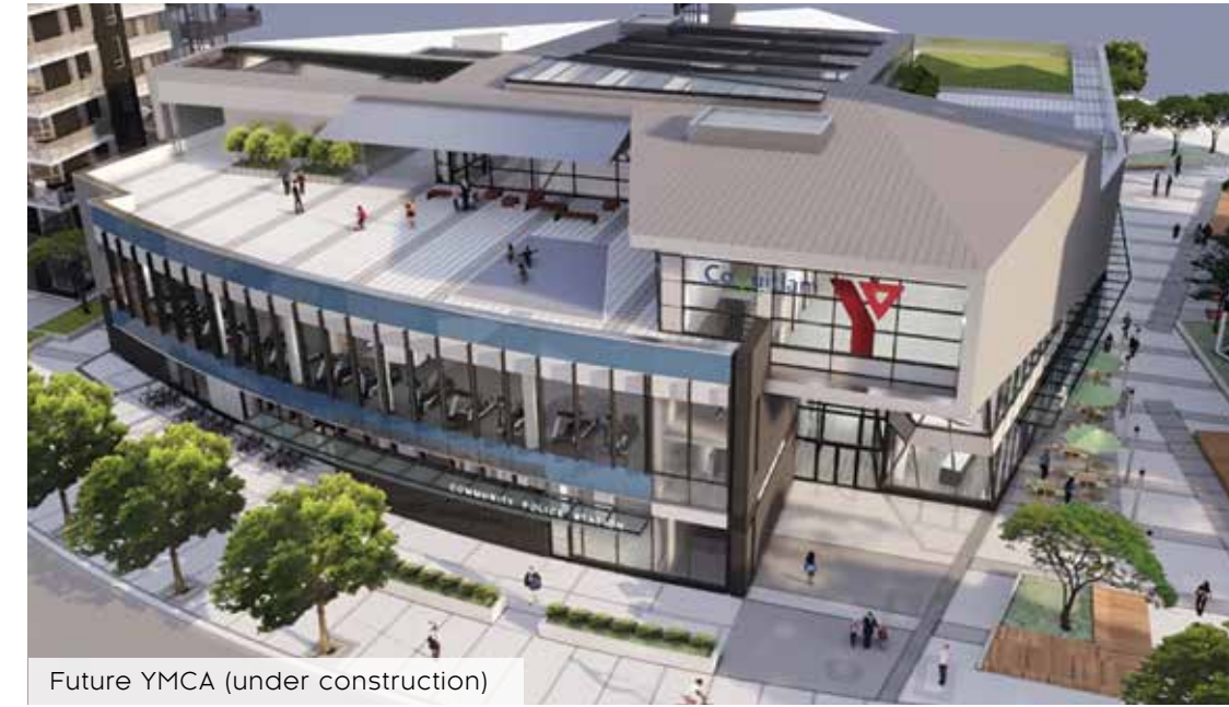
Future YMCA (under construction)
